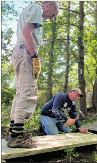
Volunteers help construct bog bridging at Smelt Brook Preserve to protect trails vulnerable to erosion.
